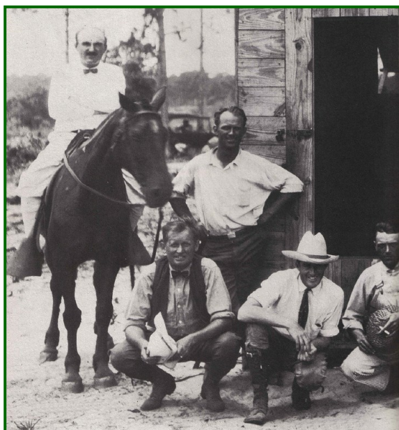
Toomey and Flynn Construction Crew Lawrence, Gordon, and Wilson
